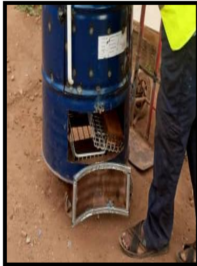
Fig 18: Laying of the firewood box bricks
