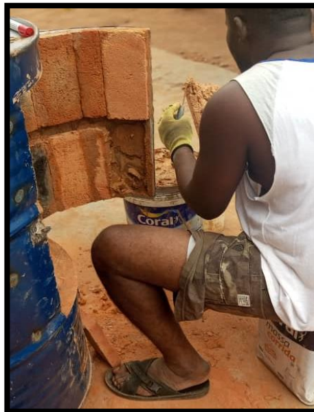
Fig. 16: Laying of the inside brick
