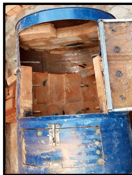
Fig. 17: Laying of the brick at the door
