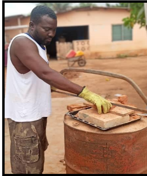
Fig. 14: Complete skeletal structure of the oven Fig. 15: Sizing of the brick by cutting
